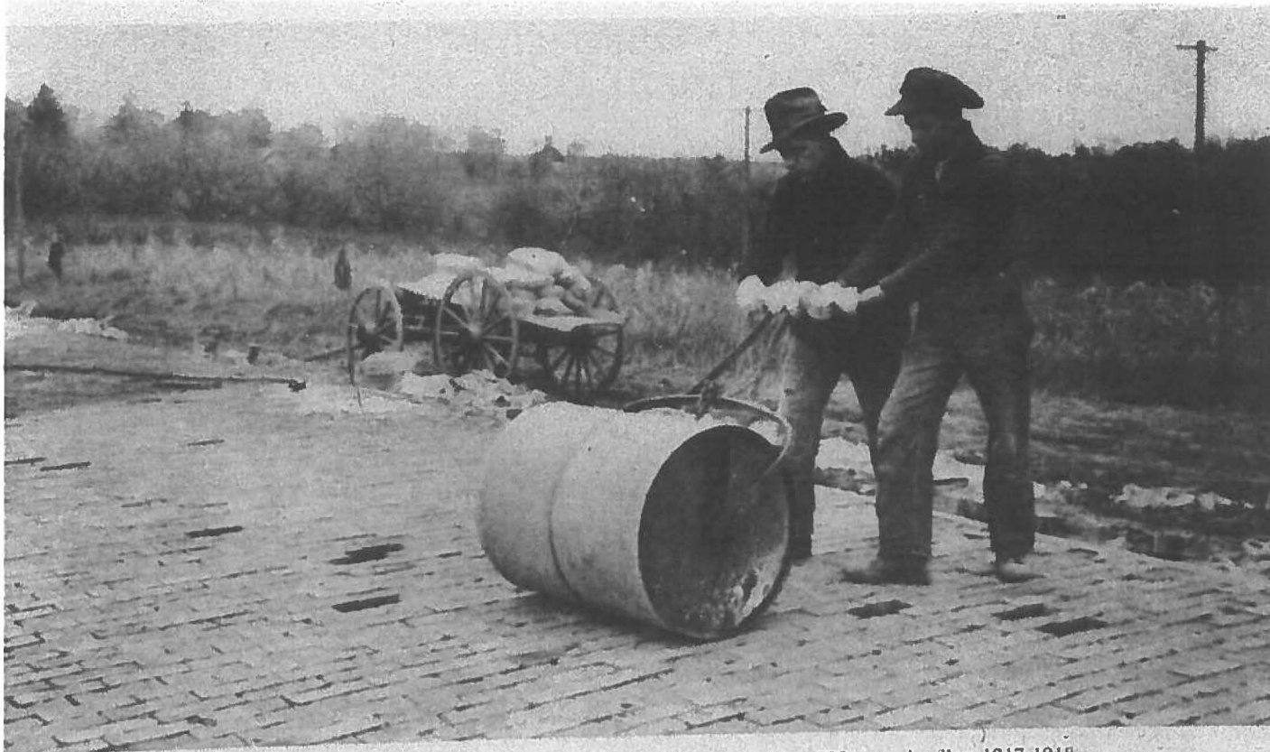
Rolling the Des Moines to Camp Dodge brick pavement with a 700 pound roller, 1917-1918 (Courtesy: Iowa State Highway Commission)
