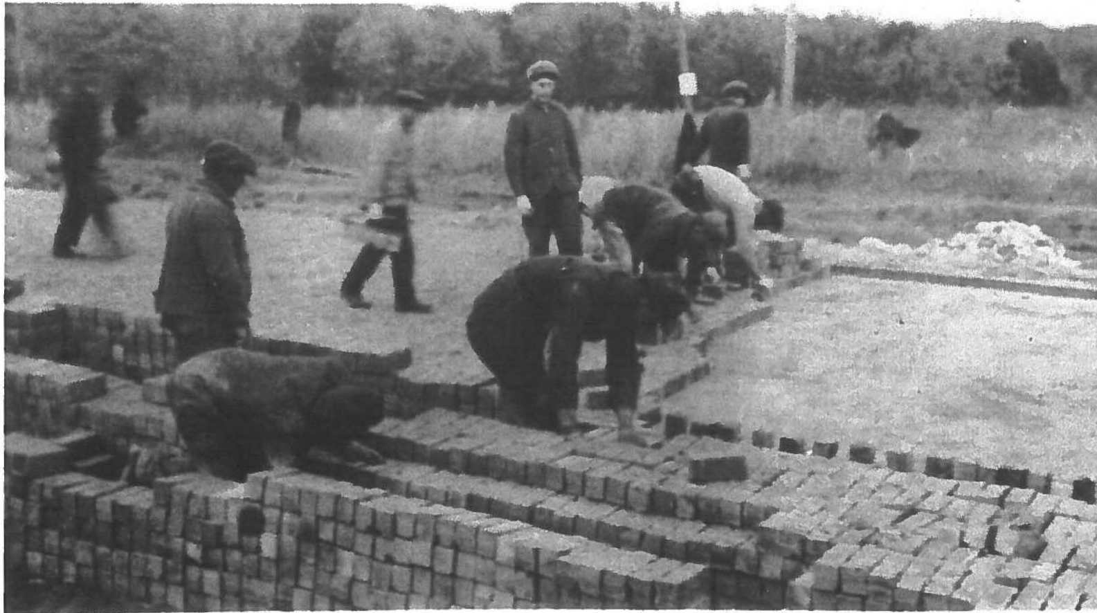
Placing monolithic brick pavement for the Des Moines to Camp Dodge road, 1917-1918. (Courtesy: Iowa State Highway Commission)
